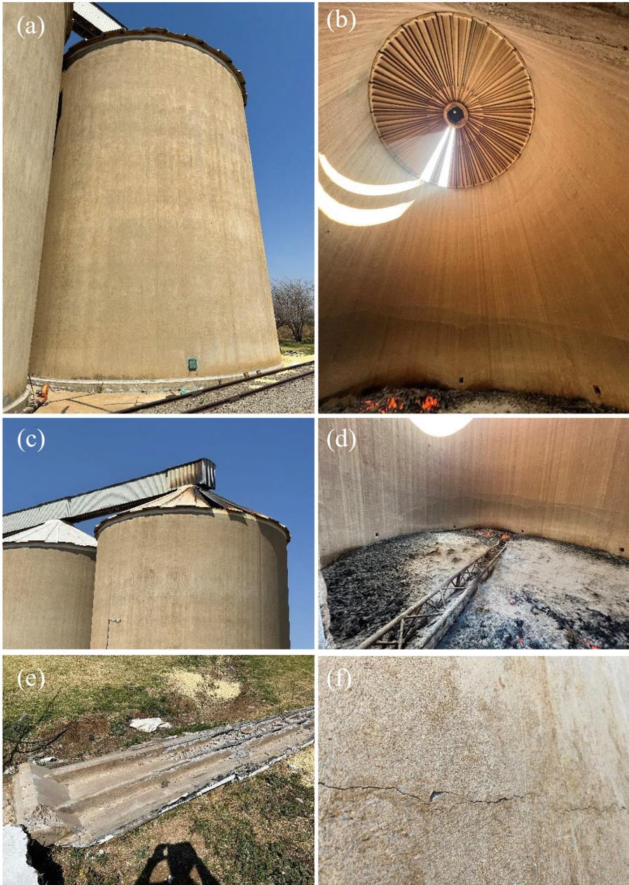
**Fig. 1.** Images of the fire damaged silo showing: (a) external view of the silo, (b) view of the roof from inside, (c) roof and transfer structure, (d) internal charred material and smoldering fire, (e) precast concrete panels which were propelled by steam off the roof, and (f) example of cracks in the walls when viewed from the outside.
